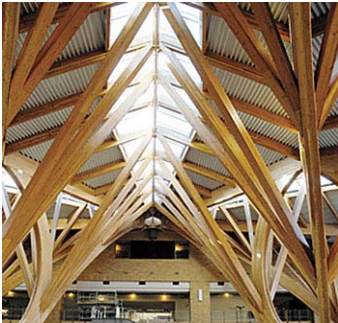
Peel Regional Cancer Centre and Ambulatory Care at the Credit Valley Hospital
