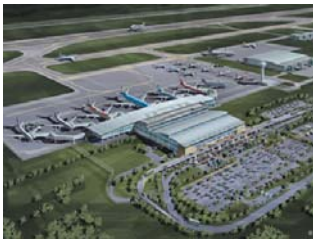
New Quito International Airport, Quito, Ecuador
